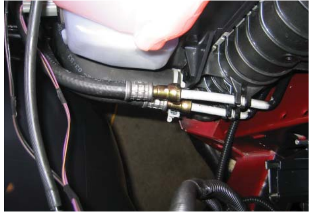
Main Water Line Clamps
